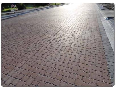
When used as part of Advanced Pavement Technology's exclusive BASS™ method, these pavers allow for natural stormwater drainage and groundwater recharge, making the paved surface ecologically sound and economically smart. In fact, the BASS™ method is an acceptable post-structural Best Management Practice (BMP) used to meet the federal stormwater management requirements. Roads and parking lots created using BASS<sup>™</sup> with these permeable pavers offer vast benefits:
